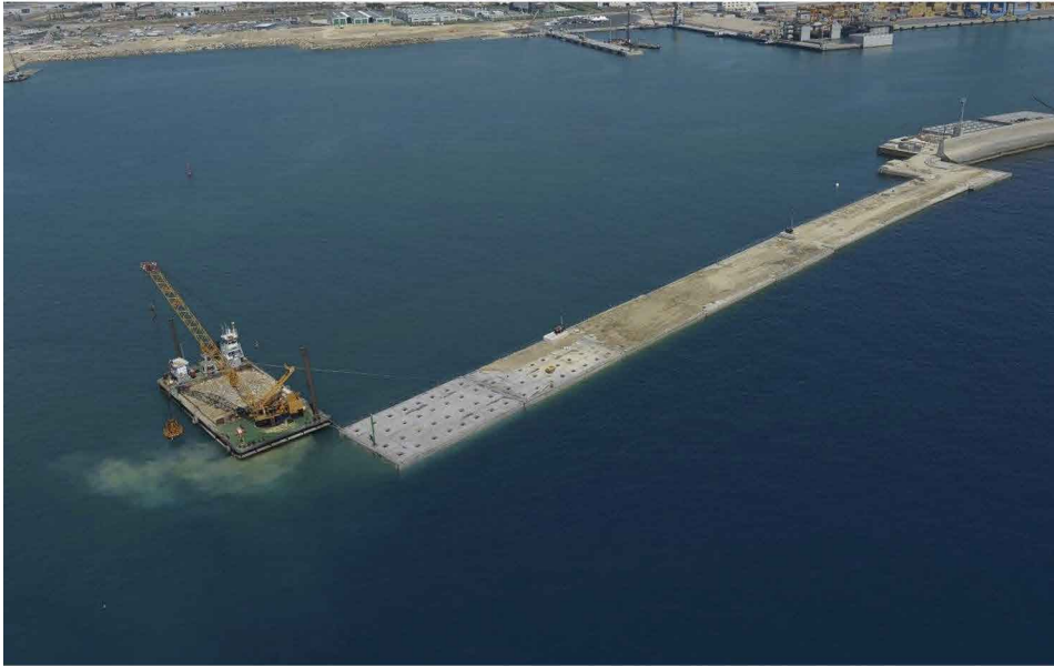
1c ROCK BERM FOUNDATION REALIZATION, POSITIONING THE CAISSON JOINED AND FILLING WITH CONCRETE
