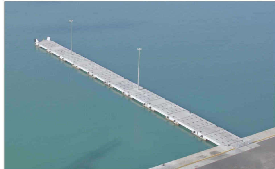
3A FINAL STEP: ELECTRICAL, LIGHTS, WATER AND FIRE FIGHTING SYSTEM INSTALLATION, FENDERS, LADDERS, BOLLARDS, RINGS
