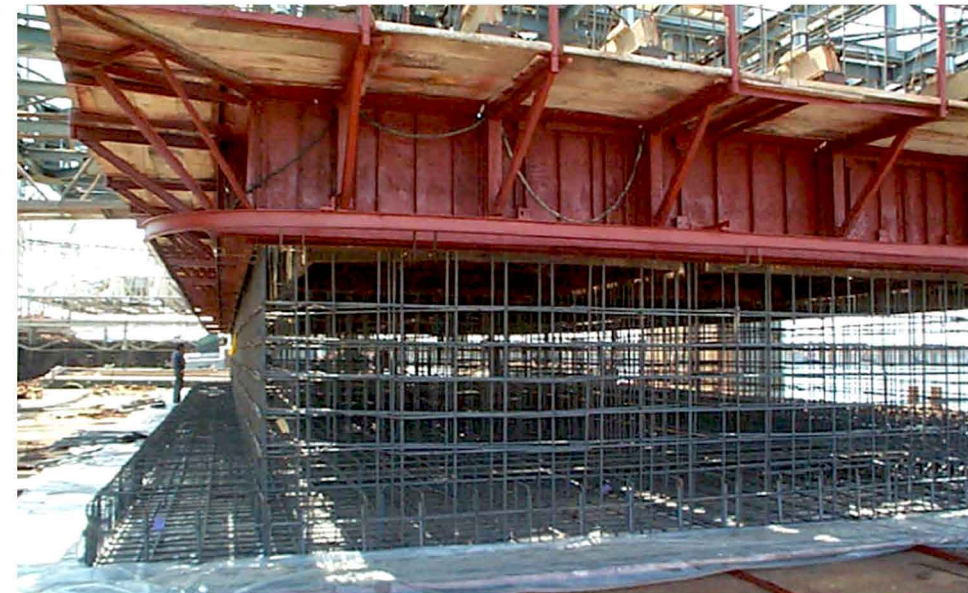
2 REINFORCEMENT CAGE: BOTTOM SLAB, INTERNAL AND EXTERNAL VERTICAL WALLS. POURING THE SLAB AS A MONOLITHIC ELEMENT
