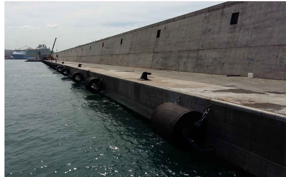
3c FINAL STEP: ELECTRICAL, LIGHTS, WATER AND FIRE FIGHTING SYSTEM INSTALLATION, FENDERS , LADDERS, BOLLARDS SETTINGS
