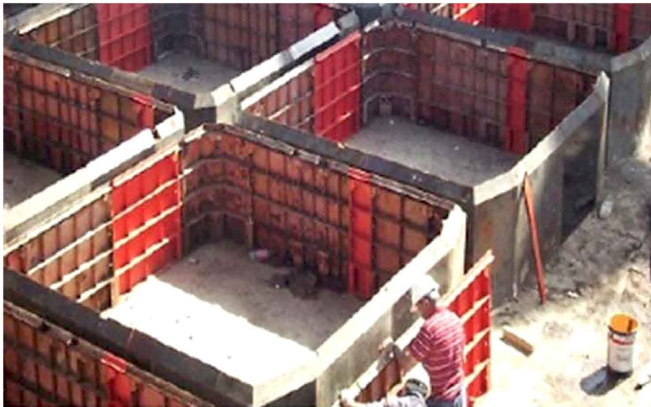
1 FORMWORK ASSEMBLY FOR INTERNAL AND EXTERNAL CELLS
