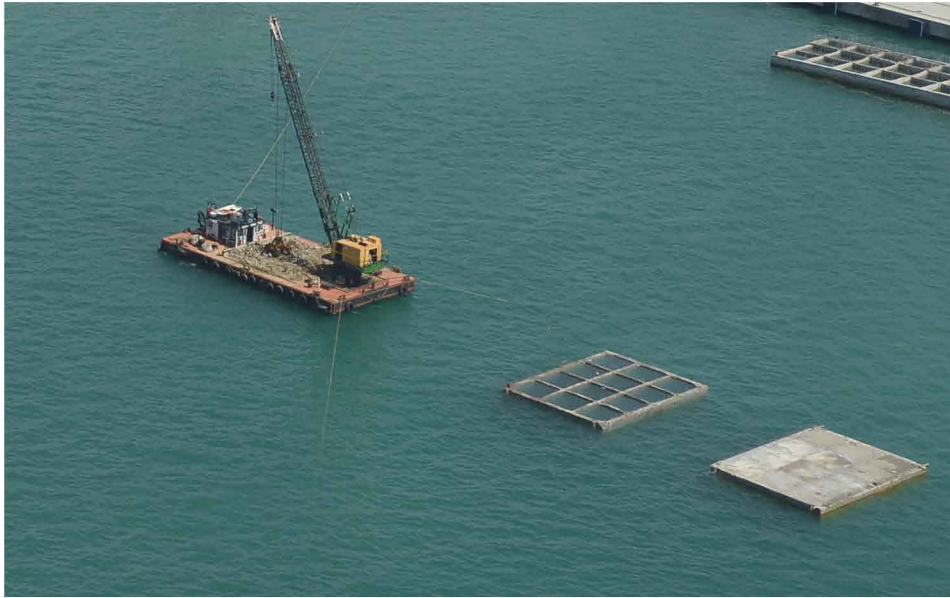
1A POSITIONING THE FLOATING CAISSON FOR THE JETTY
