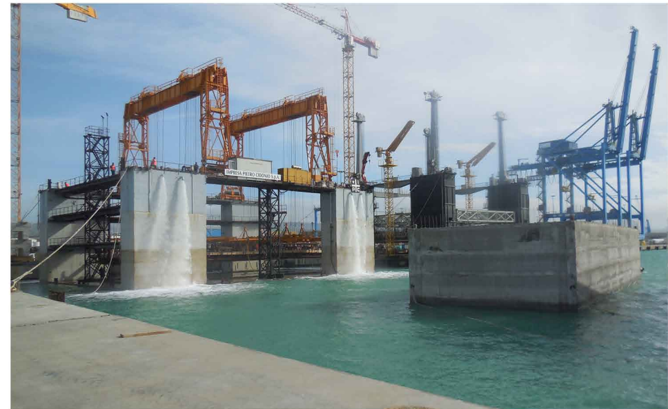
6 AT THE END OF THE CONSTRUCTION PHASE, THE PLATFORM WERE SLID DOWN TO ALLOW THE LAUNCHING FROM THE DOCK
