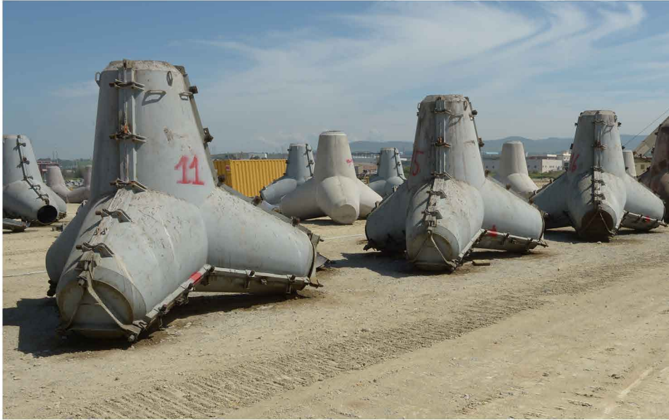
1 TETRAPOD BLOCKS: TETRAHEDRAL PRECASTED CONCRETE STRUCTURE DESIGNED TO DISSIPATE THE FORCE OF THE WAVES
