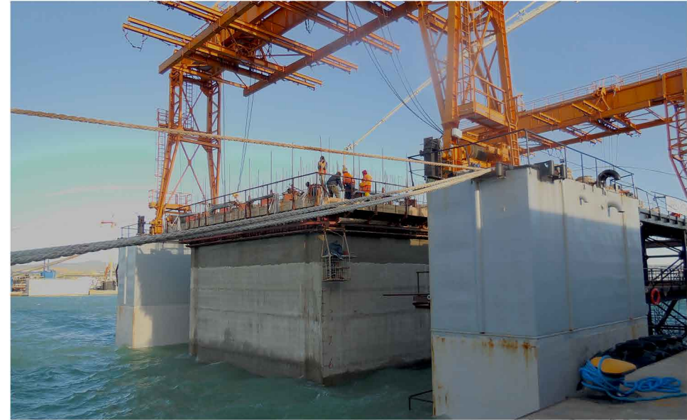
5 SEQUENCES 3-4 WERE REPEATED UNTIL THE TOTAL HEIGHT OF THE CAISSON WAS REACHED
