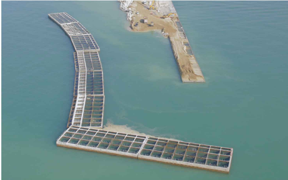
1B ROCK BERM FOUNDATION, I POSITIONING THE CAISSON JOINED, FILLING CONCRETE, GRAVEL BACKFILL SETTINGS, EMBANKMENT
