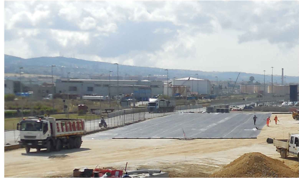
3 TERMINAL PAVEMENTS REALIZATION WITH A BEARING CAPACITY OF 10 t/MQ
