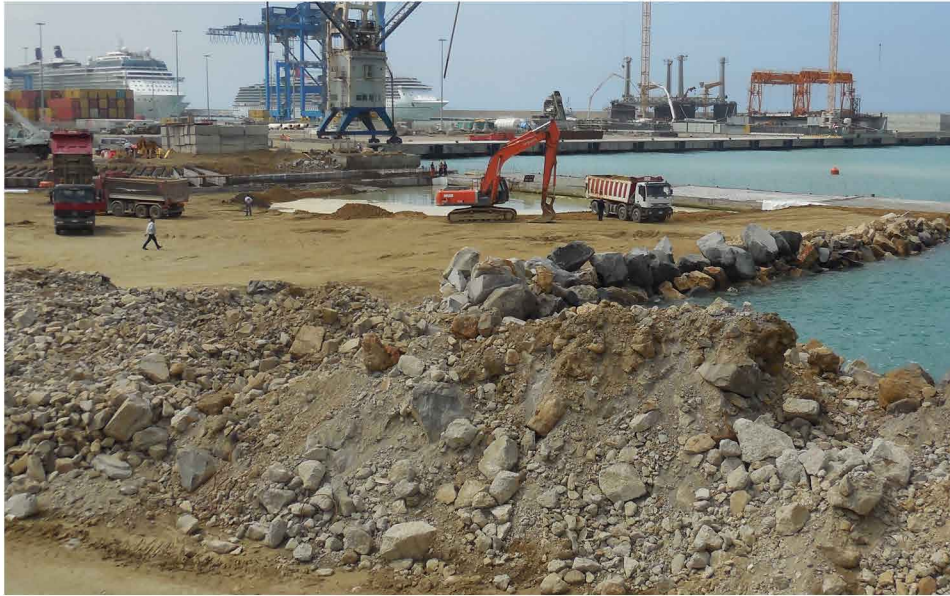
1 LAND RECLAMATION: EMBANKMENT FILL WITH DREDGED SOIL
