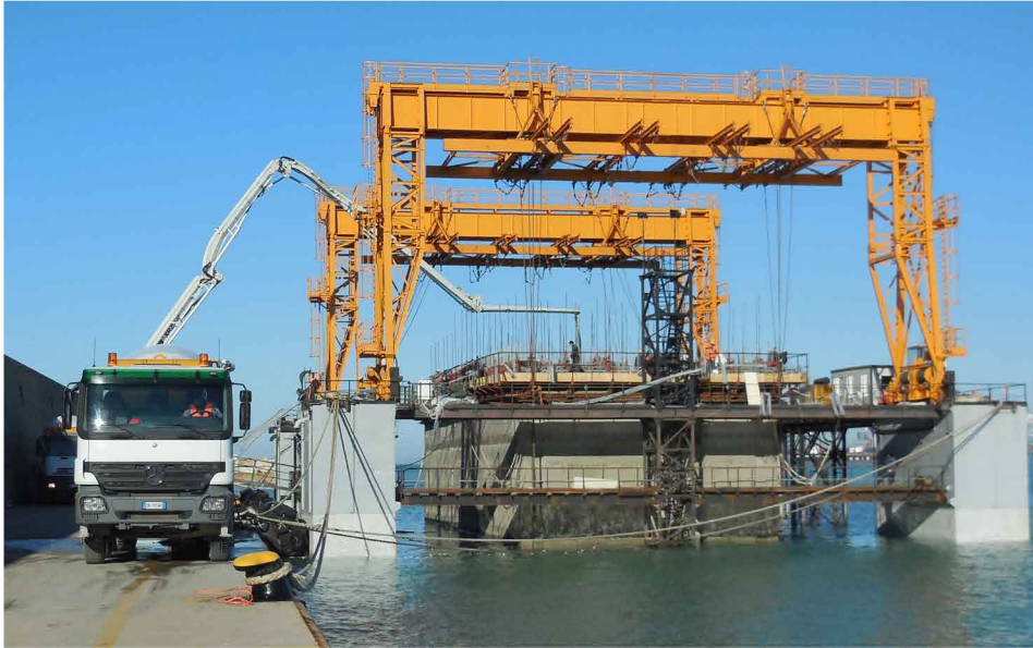
THE FLOATING CAISSONS ARE CONCRETE BOX WITH CELLES, THEY WERE PREFABRICATED USING THREE SPECIAL FLOATING DOCKS
