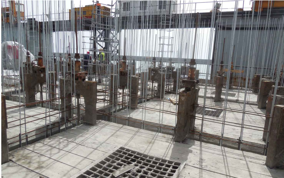
3 PLACING THE REINFORCEMENT, UNDER THE CONTROL OF THE CONSTRUCTION SUPERVISOR
