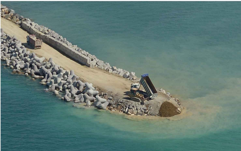
2 CONSTRUCTION OF THE BREAKWATER CORE WITH DREDGING MATERIALS AND THE PROTECTION LAYERS WITH TETRAPODS
